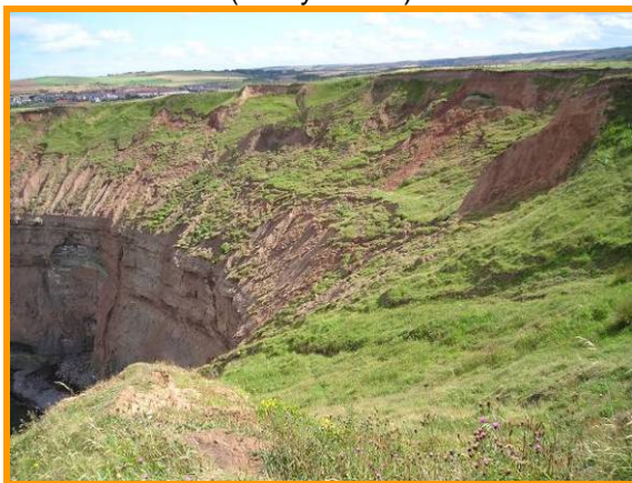
E59/5 failure and active headscarp recession within the upper till part of the cliff (Partly Active)
