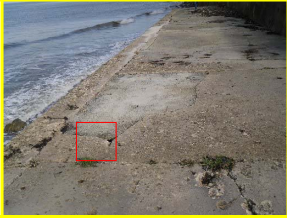
Top of wall with void location indicated (Asset Ref No. 1221D901D0202C03)
