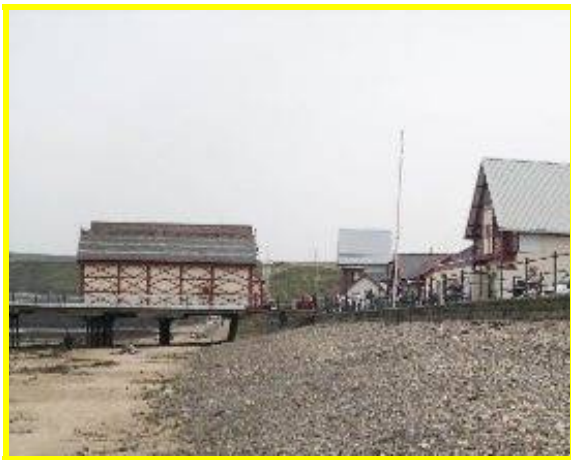
View of pier and sea wall. (Asset Ref No 1221C901C0704C04)
