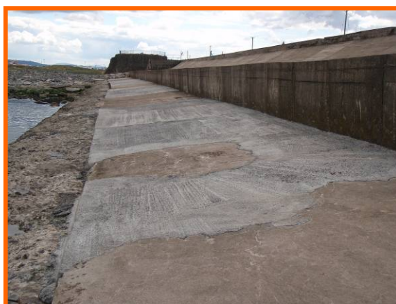
Slab repairs to deck on east side of structure – 2010 (Asset Ref No 12221C901C0506C01)
