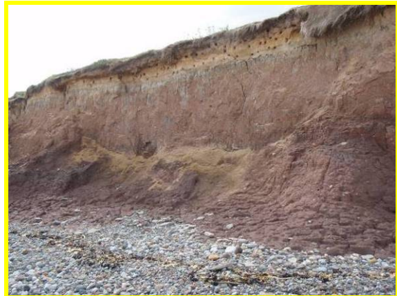
E52/10 Local headscarp failure (Locally Active)
