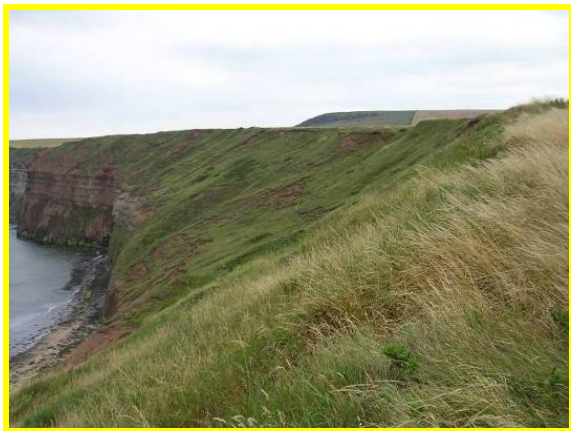
E53/4 Slumping in the till layer of the cliff northeast of Saltburn (Locally Active)
