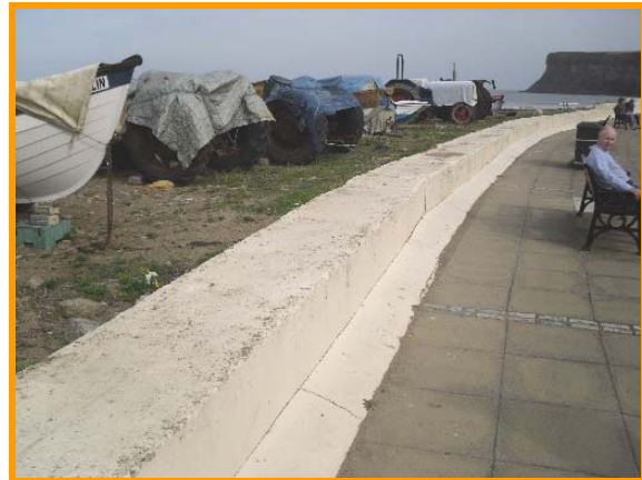
View of sea wall (Asset Ref No. 1221C901C0704C03)
