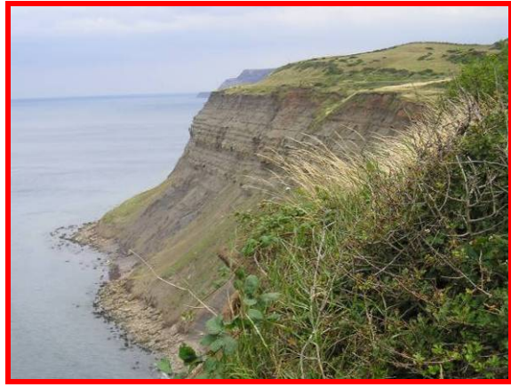
E54/3b looking southeast along Warsett Hill (Totally Active)
