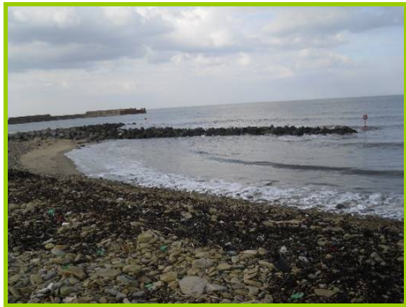
Fishtail breakwater (Asset Ref No. 1221D901D0202C05)
