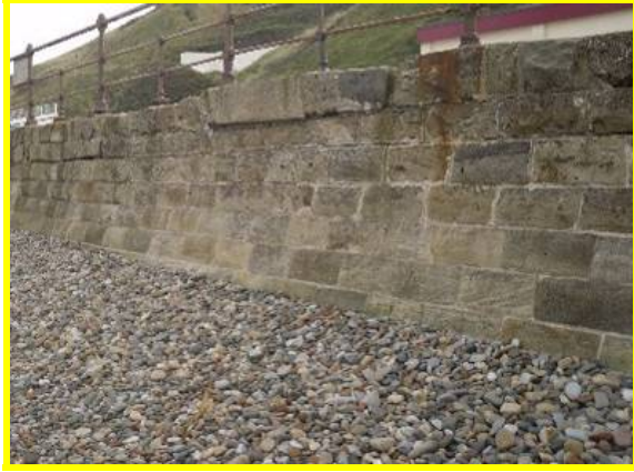
Example of coping repair (Asset Ref No 1221C901C0704C04)
