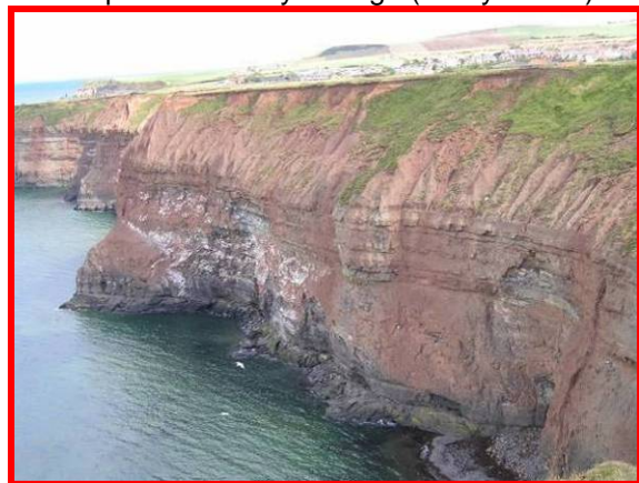
E59/4 fresh failures within the till and rockfall from lower cliff face (Totally Active) (Note: this unit was previously classified as Partly Active in 2008)
