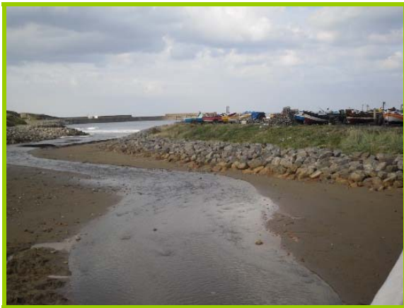
Fishtail breakwater (Asset Ref No. 1221D901D0202C05)
