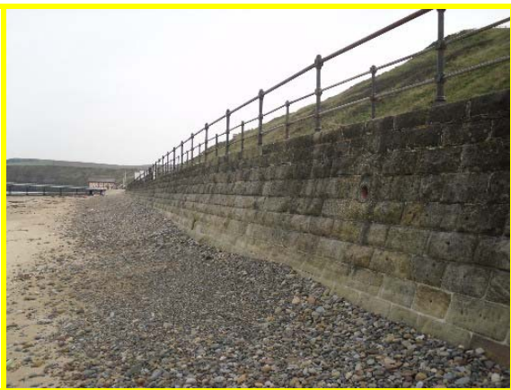
View looking east along Lower Promenade (Asset Ref No 1221C901C0704C04)
