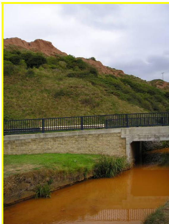
E52/1 erosion at the head of the mound just east of Saltburn Gill (Locally Active)
