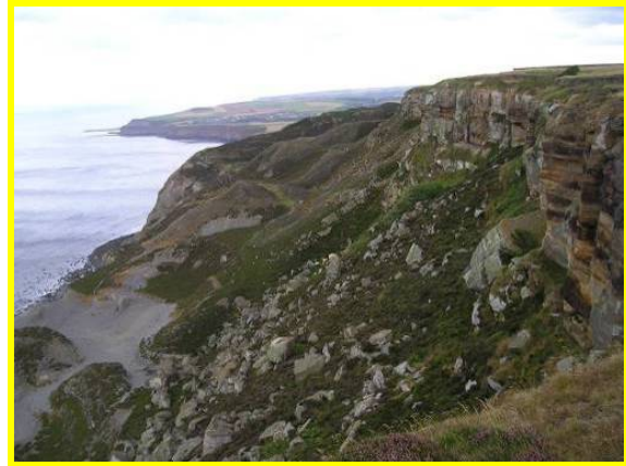
E58/2upper evidence of past rockfall (Locally Active)
