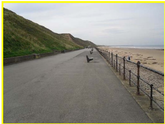
View looking west along Lower Promenade (Asset Ref No 1221C901C0704C04)
