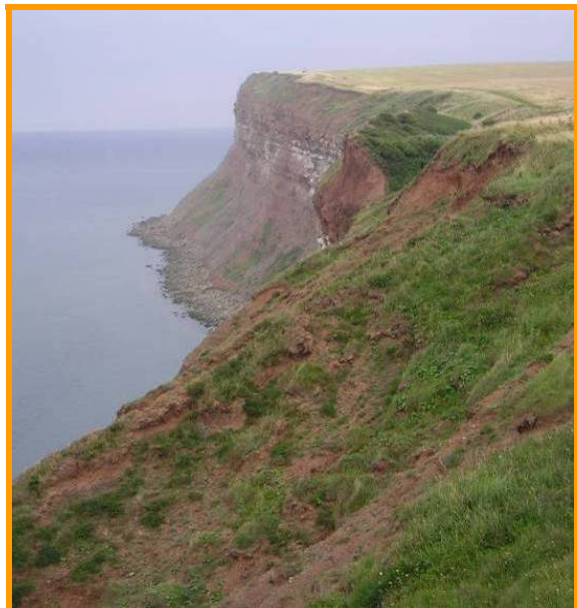
E53/2 Lower debris cones and staining of the cliff in the distance (Partly Active)
