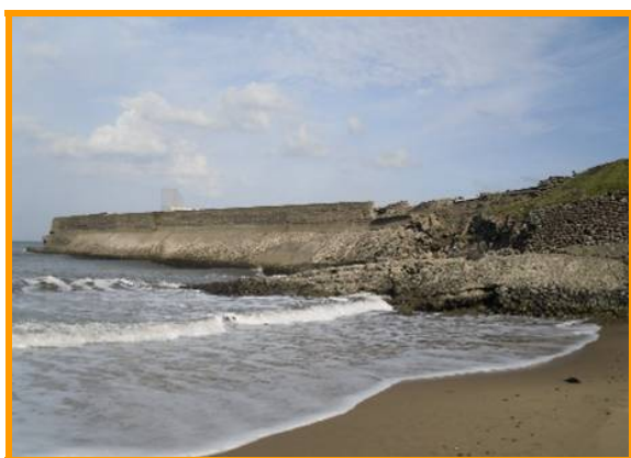
Jetty – view from NW side (Asset Ref No. 1221D901D0201C02)
