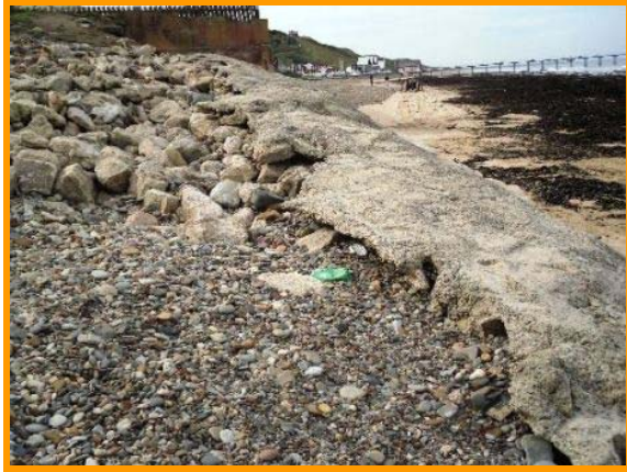
2010: View of repairs – mass concrete and rubble (Asset Ref No. 1221C901C0704C05)
